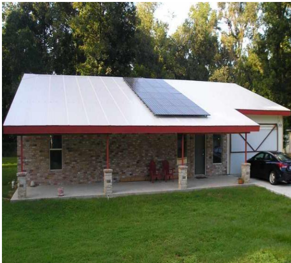
5 kw Solar, - 450$ annual energy cost
